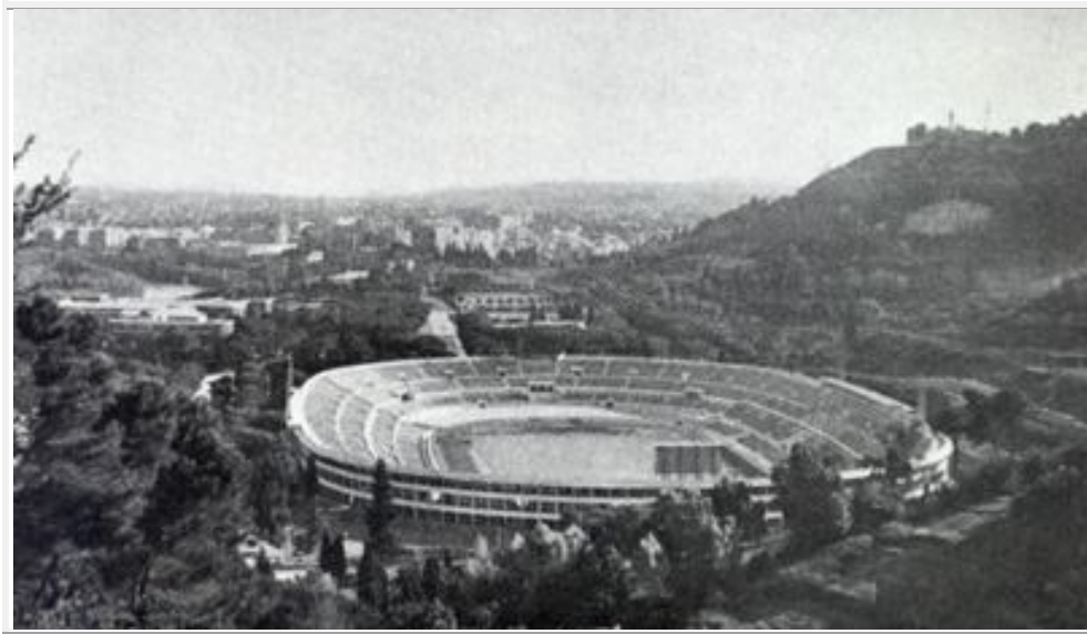
1960 Rome Olympic Stadium
